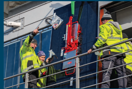
Montage des BIPVslim Systems an die Fassade des Energy Efficiency Centers.
